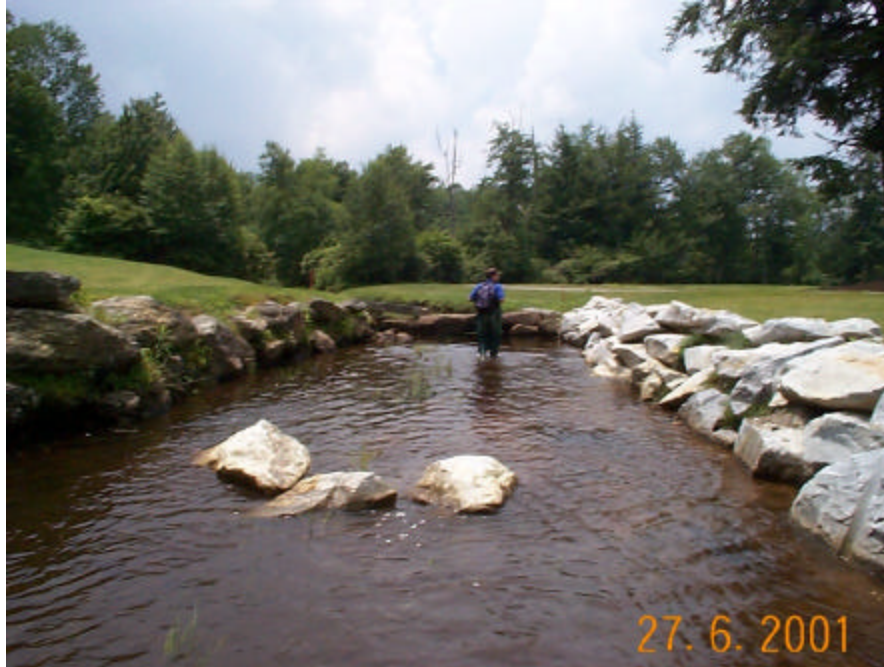
Figure C.3. Riprapped banks on the Cullasaja River in a golf course.
