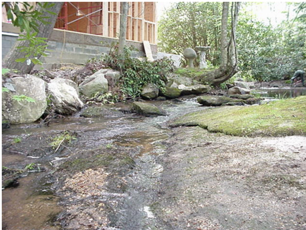
Figure 7.1 Construction of house on Mill Creek at 5 th Avenue.
