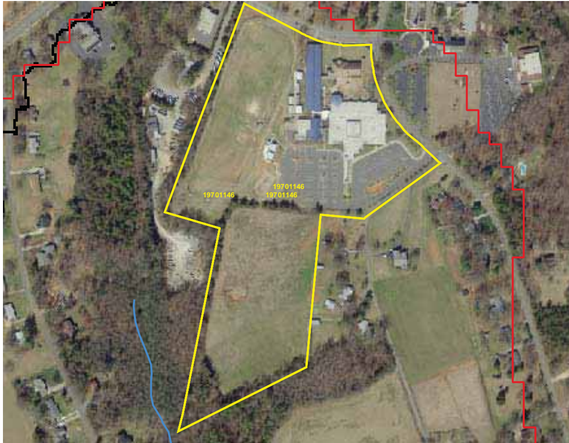
Figure 31: Aerial Photo of Parcel 19701146 (Medium Priority).
