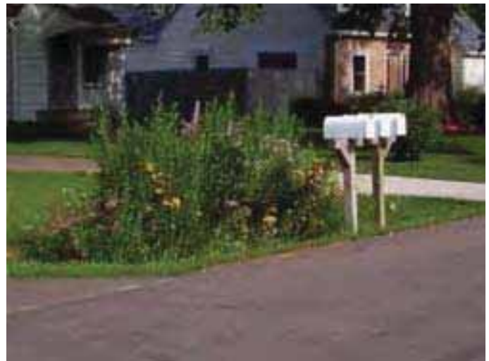
Photo: Bioretention cells look like simple, aesthetically pleasing plantings from the casual observer, however, they are only the visible topping of a 2-3 foot porous medium installed directly below. The exact size and capacity of these structures are engineered based on the intensity and duration of rain events in the study area. Low Impact Development Center, Inc.
