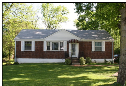
An example of a Transitional Ranch house, ca. 1955, in the Inglewood Place Historic District
