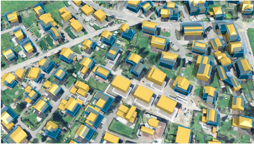
Figure 10.1: Two datasets of different LODs of the same area but of different lineage. The models (LOD1 and LOD2) are produced in separate campaigns, resulting in different positional accuracies and varying completeness. 31
