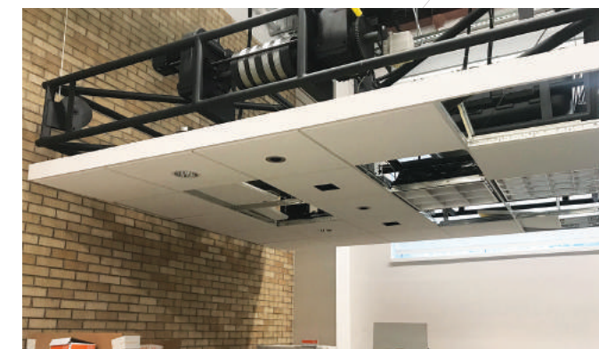
The FAB’s lighting lab has an operable ceiling that students can use to simulate commercial and residential ceiling heights when working on lighting projects. The design of the ceiling is flexible to easily change the light fixtures as technology advances.
