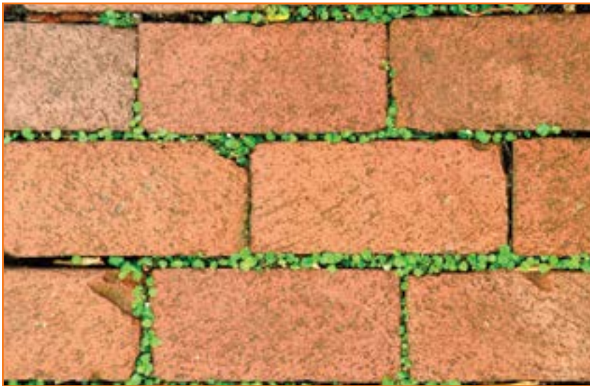
Figure 29.2 Lawn pennywort ( Hydrocotyle sibthorpioides ) in sidewalk cracks in front of our row house in Center City. The plant leafs out, blooms, makes seed, and spreads entirely within these cracks, which protect it from trampling. A creeping perennial introduced as an ornamental from Asia, it was first reported naturalized in Philadelphia in 1909. 4
