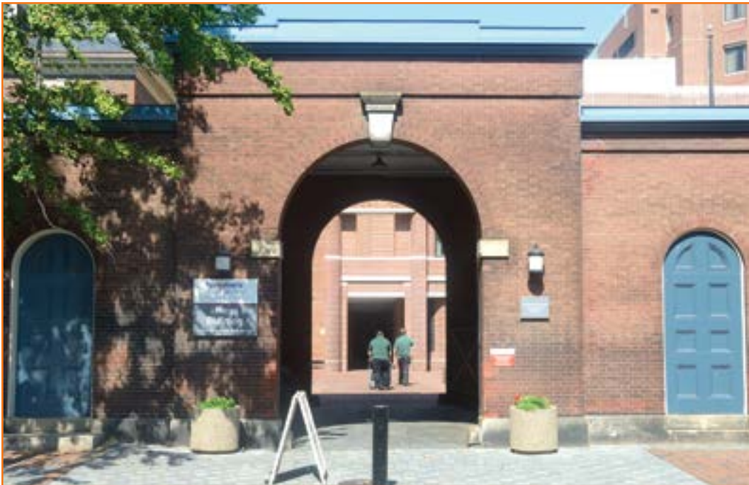
Figure 10.3 Arched entrance to Pennsylvania Hospital from 8th Street. A mud dauber is constructing her nest inside the archway.
