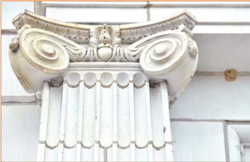
Figure 10.9 Close-up view of figure 10.8. Mud dauber nest is the brown structure on the right.
