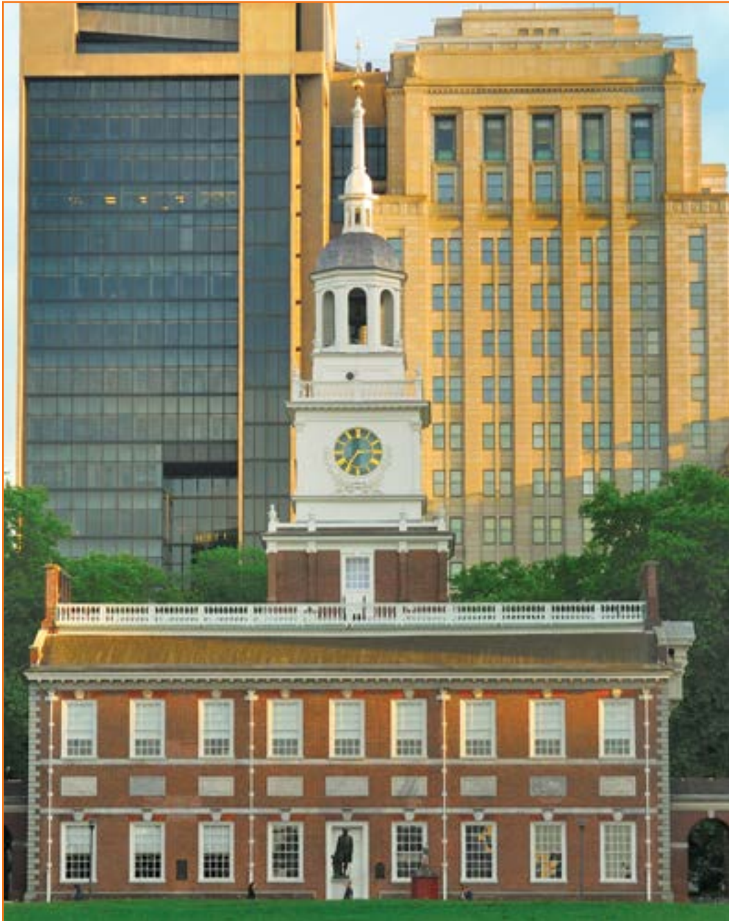
Figure 1.3 Independence Hall, constructed with bricks made from clay deposited a few blocks away by glacial meltwater.
