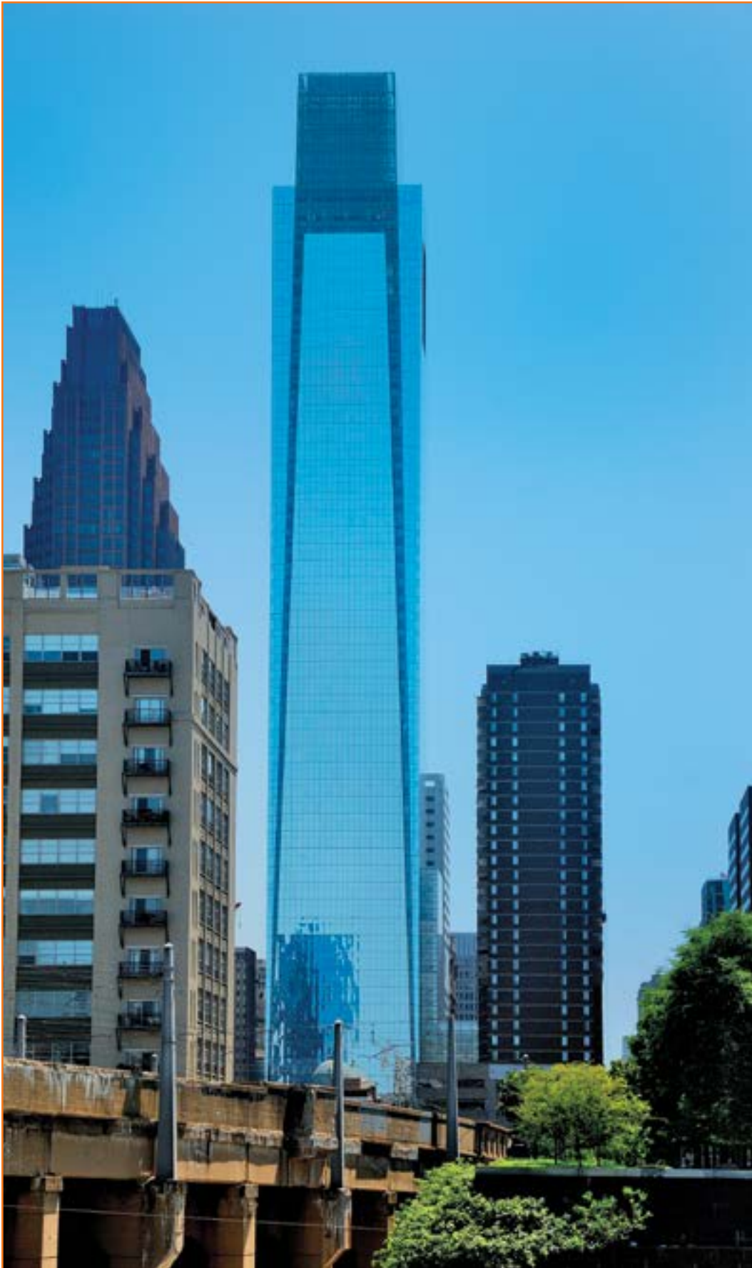
Figure 7.3 Comcast Center's glass façade blending in with the sky. One thousand birds per year have been estimated to die striking this and adjacent buildings.
