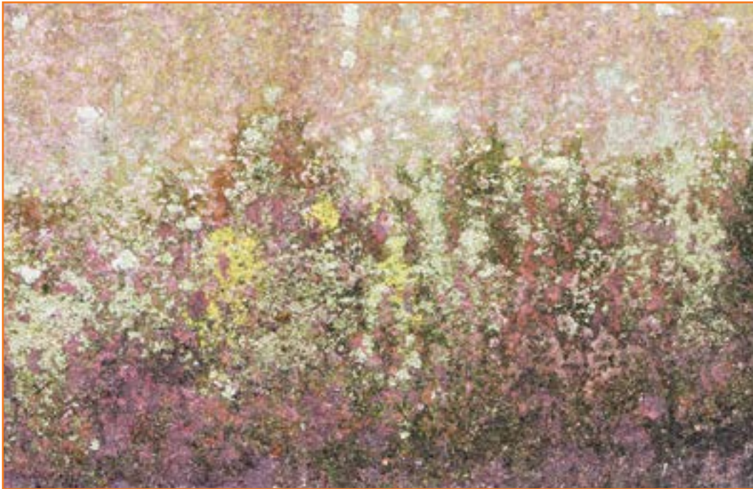
Figure 23.14 Lichens covering stucco on rear wall of South Square Market, which fronts on South Street. Air pollution suppresses the diversity of lichens, but some lichens thrive in it.
