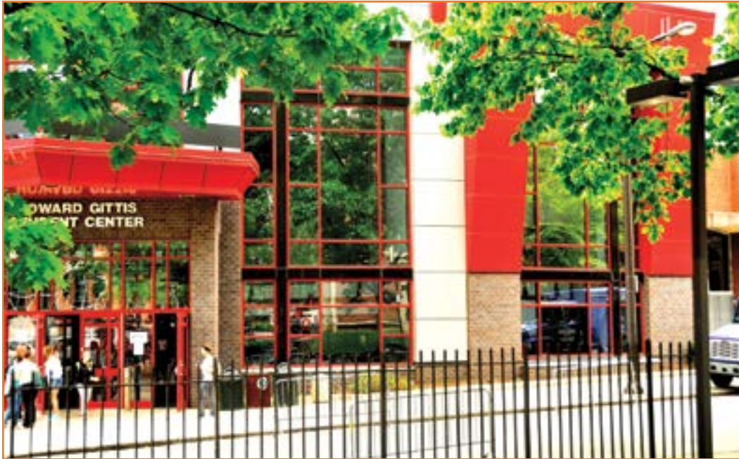
Figure 7.5 Temple University's Howard Gittis Student Center, with windows that reflect images of street trees, promoting collisions by birds. In 2011, 1,200 birds including thirty-one species were recovered around Temple's campus buildings, including this building.
