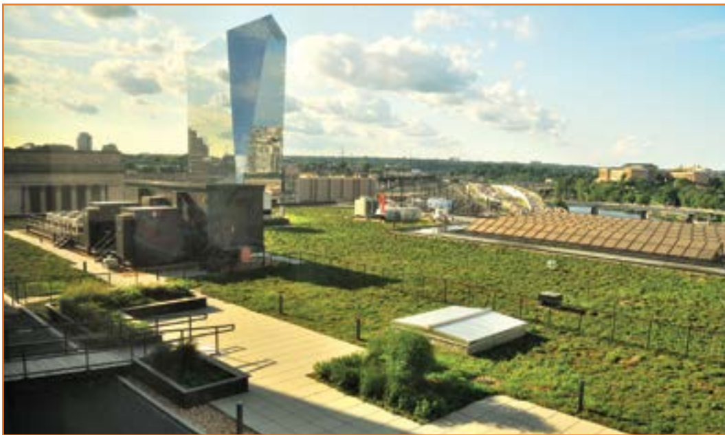
Figure 29.3 Green roof on top of PECO (Philadelphia Electric Company) building in Center City.
