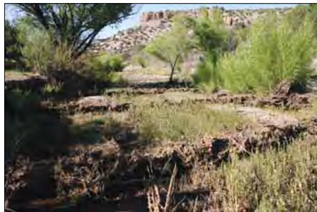
Fig. 3. Step-down-woven-weir slows water, captures sediment and raises cienaga bed.
