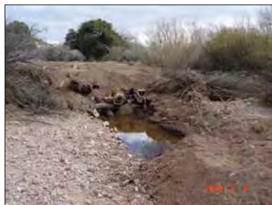
Fig. 5. Engineered logjam plugs eroded channel, elevates cienaga bed, moves water rightward to reconnect with historic waterway.
