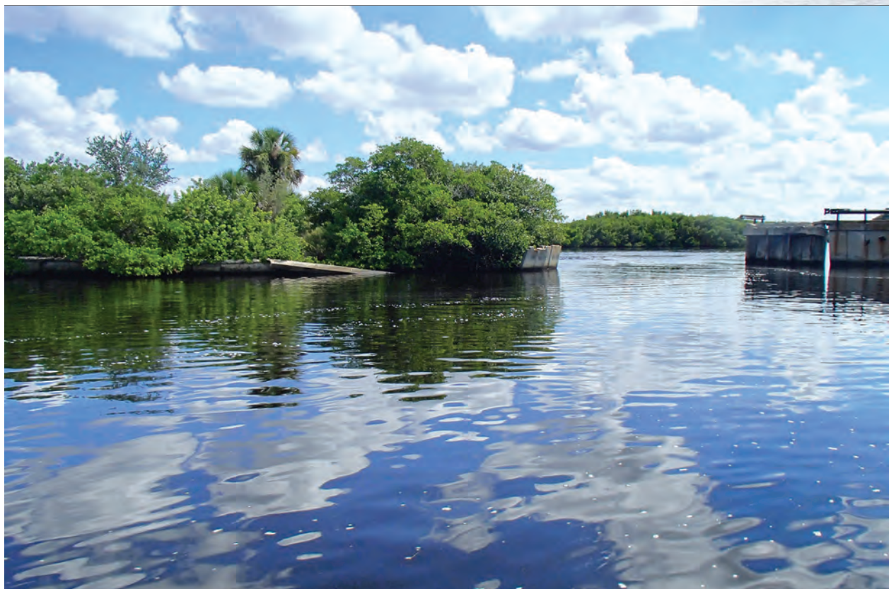
Remnants of the old Goat Island bridge detract from the aquatic preserve's natural beauty, and are a hazard to boaters.
