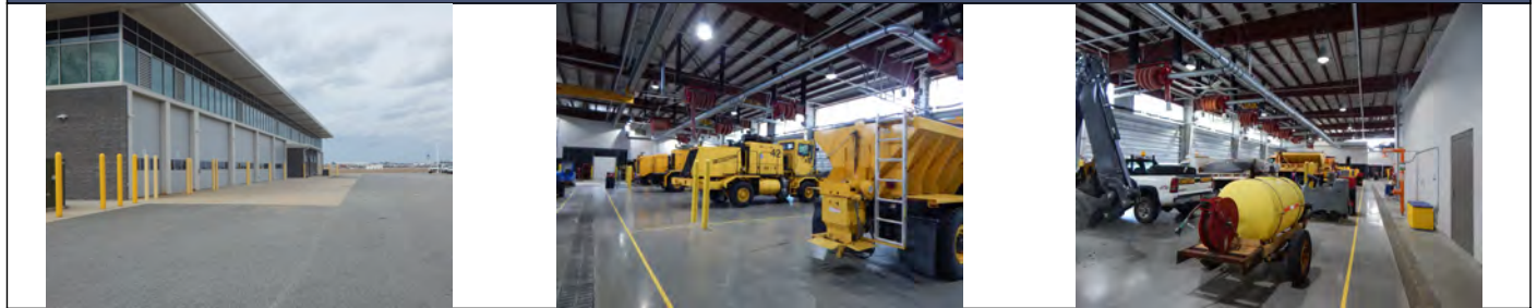
*Building Conditions: Good (10+ Years); Fair (5-9 Years); Poor (1-4 Years) *Square Foot Measurements are Estimates
