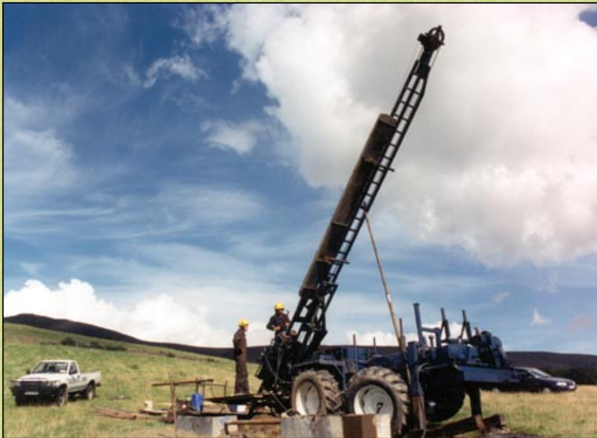
Above: Drilling rig at Rhynie during the summer of 1997.
