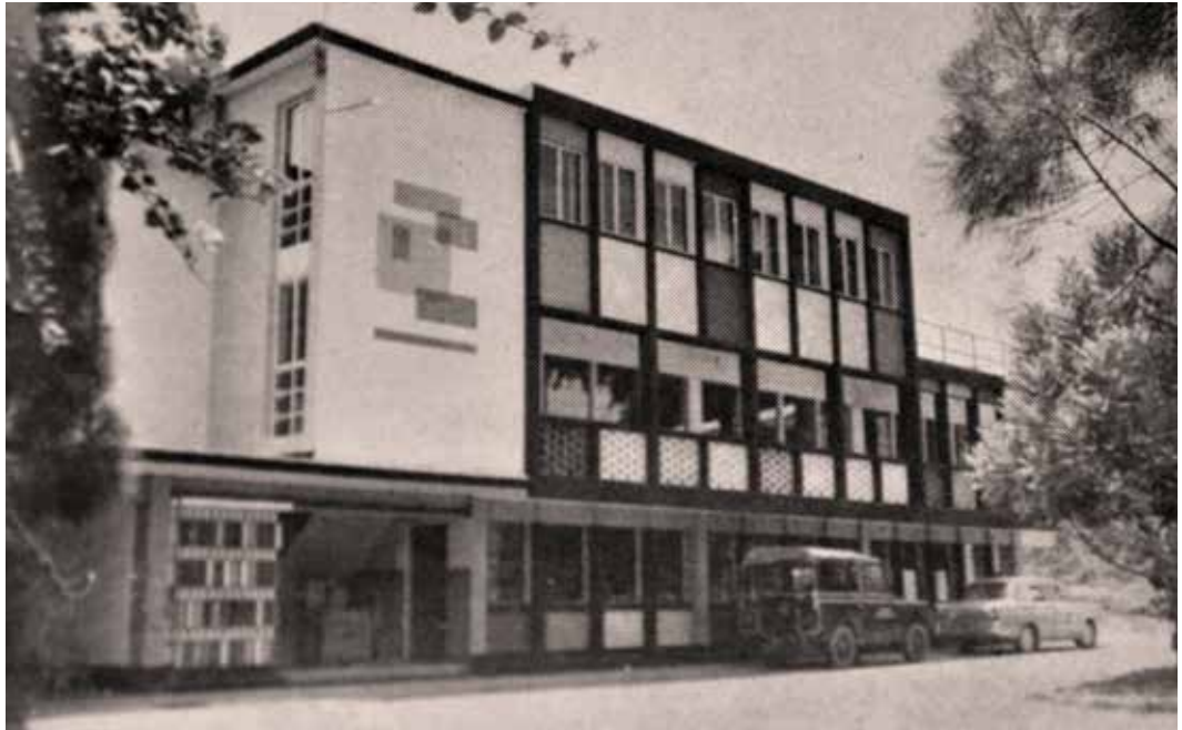
Fig. 4. The Sandakan Herbarium was housed in a building on the Ching Meng School premises in 1964. (Forest Research Centre archives)
