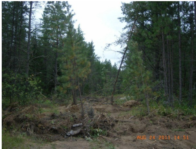
Figure 2-1: Effective road closure. Picture was taken immediately after decommissioning following a recent timber sale. Multiple berms and tree transplants were used. There was no RMV use.
