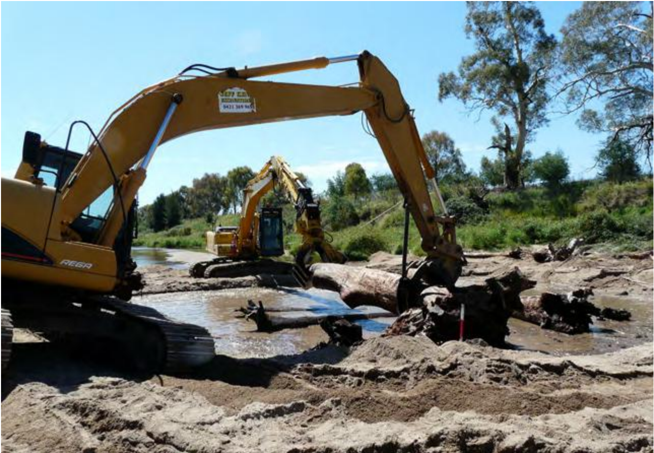
Figure 5.5 Installing log jams
