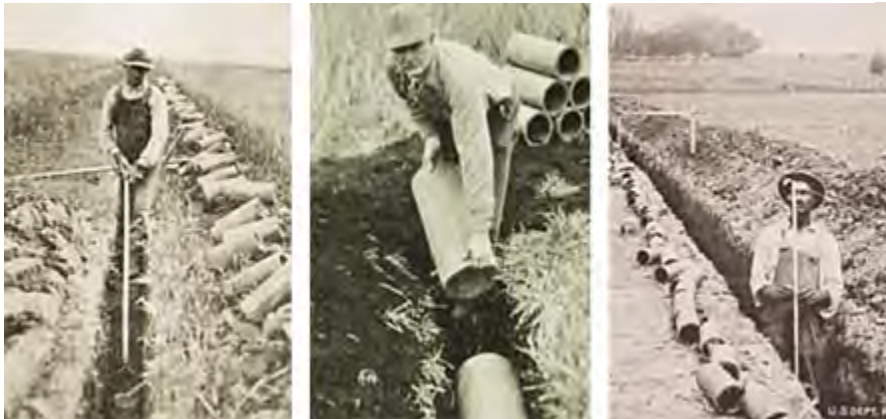
Figure 7: Tile Drain Installation
