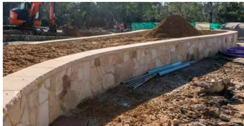
Recently completed sandstone wall
