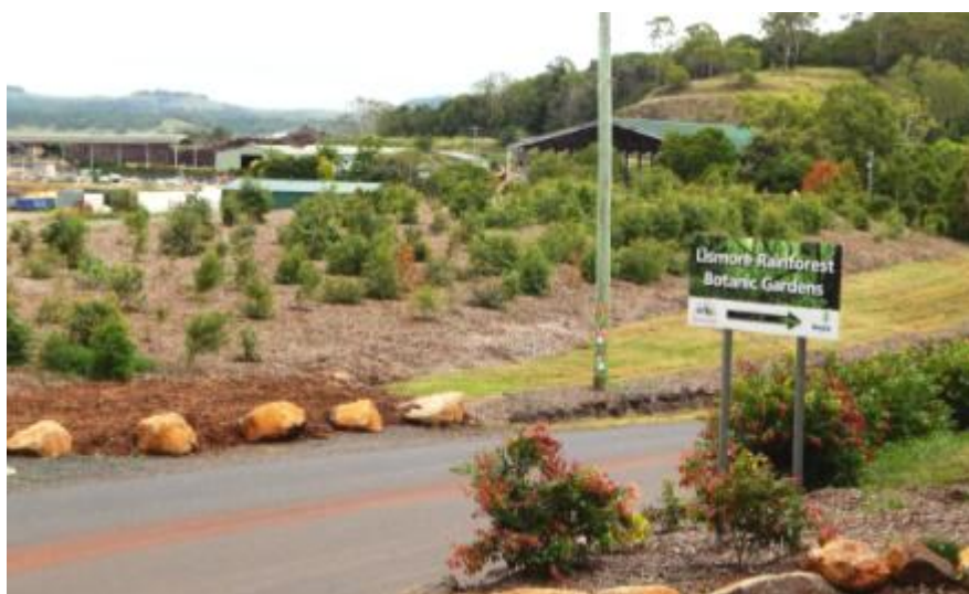
Recent phytocapping planting viewed from Botanic Gardens entrance with operational area of Lismore Recycle and Recovery Centre in the background
