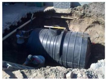
Figure 51. Underground water conservancy tank being installed.
