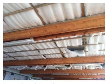
Figure 47. Ceiling insulation work in progress.
