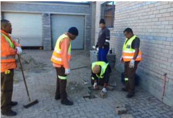
Figure 52. Paving being repaired.
