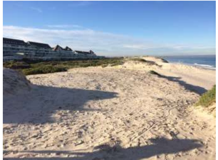
Figure 34. Extent and location of the damaged dunes in front of the Blowfish Restaurant.
