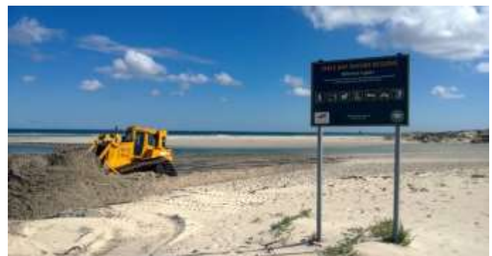
Figure 29. Stormwater machines working in lagoon mouth.
