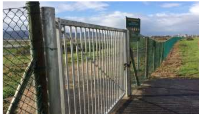
Figure 59. R27 fence at Rietvlei & CRF gate.
