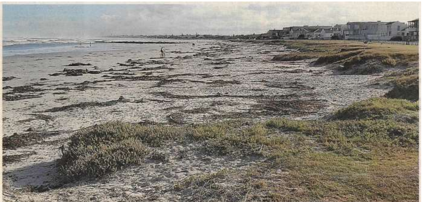
Kelp, often seen as a nuisance for beach-goers, plays a vital role in dune preservation. The removal of it is contributing to coastal erosion in Melkbosstrand.
