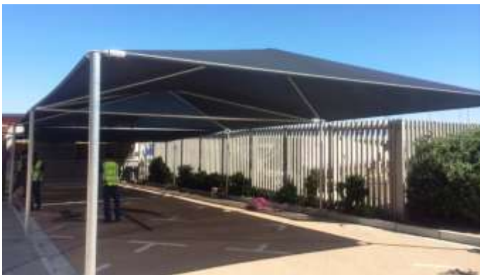
Figure 56. Office parking shadeports.
