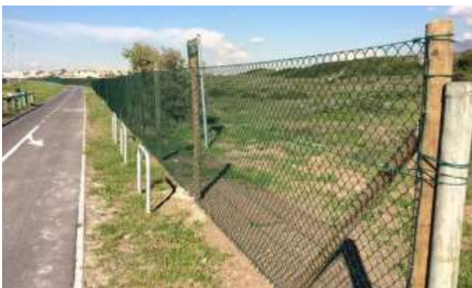
Figure 60. R27 fence at Coastal Section.
