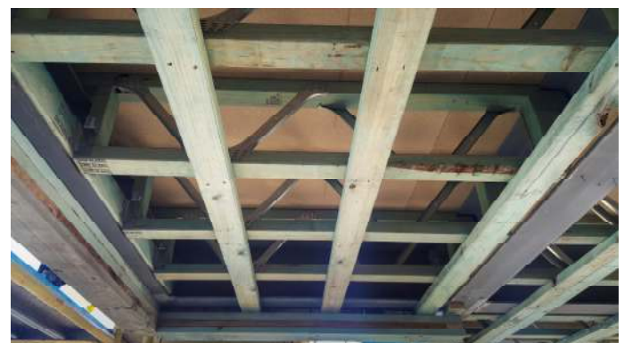
Figure 3: Floor trusses fitted in between steel beams
