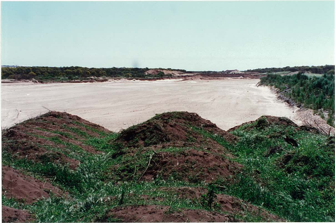
View to the North - West along the mining direction. In the foreground is stockpiled topsoil ready to be spread over the backfilled area in the middle of the photograph. The mine pit is in the middle distance.
