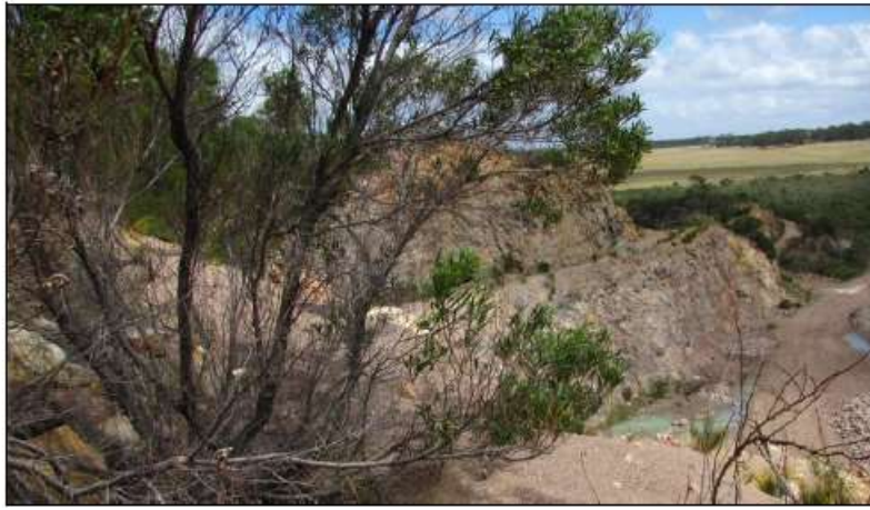
Figure 10 - Photograph includes an old bench mid-way up the quarry face (middle distance). Native vegetation in good (Keighery, 1994) condition has rehabilitated on the bench.
