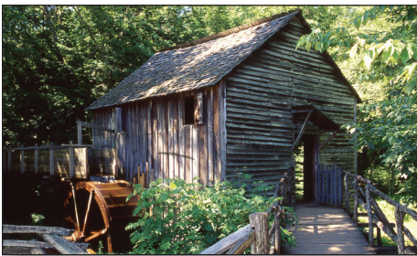
Figure 4. John Cable Grist Mill with flume and wooden water-powered wheel with 40-wheel-buckets on left side of mill and wooden walk-way to entrance.
