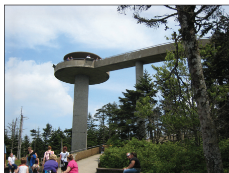
Figure 23. Clingmans Dome observation tower.
