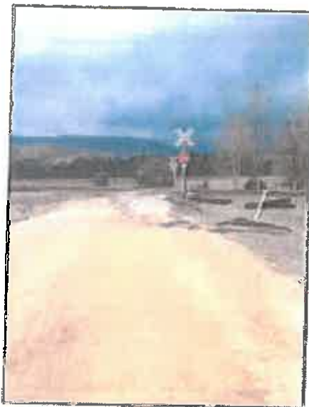
View of the railroad crossing at Canoe Creek Road.
