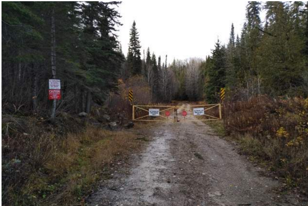
FIGURE 5.1 ACCESS ROAD PHOTOGRAPH
