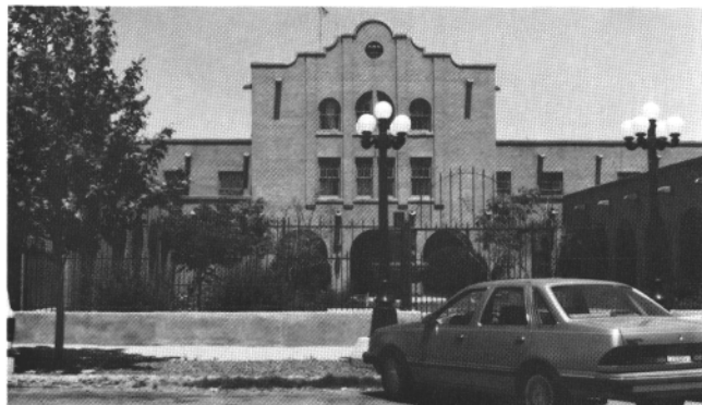
FIGURE 4—Val Verde Hotel on Manzanares Avenue, looking north.
