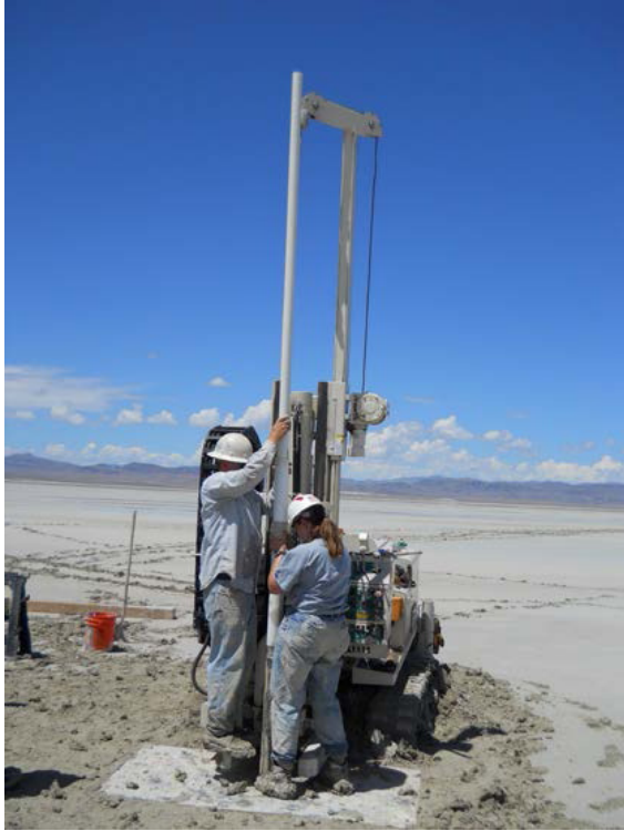
FIGURE 10-2 Photo of Direct-Push Hole Casing Installation
