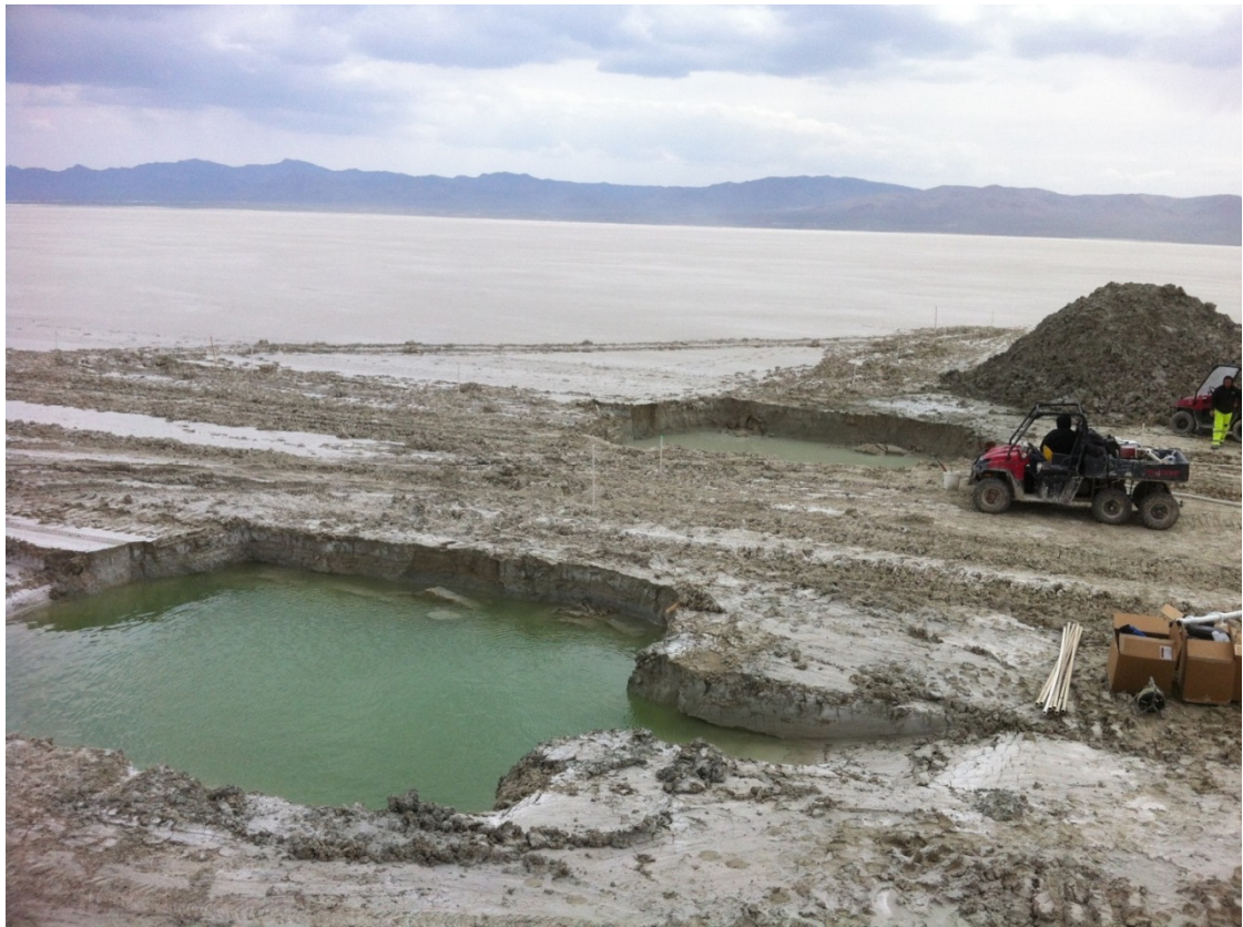
Figure 13. Photograph of Test Trench Site.
