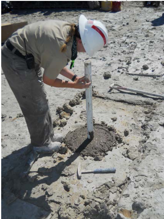
FIGURE 10-3 Photo of Direct-Push Hole Casing Completion
