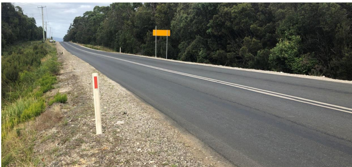
Photo 6.3B – View for drivers looking right of approaching vehicles from Bridport.
