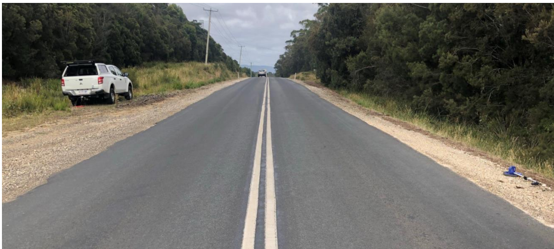
Photo 6.3 A – View for drivers looking left of approaching vehicles from East Tamar Highway
