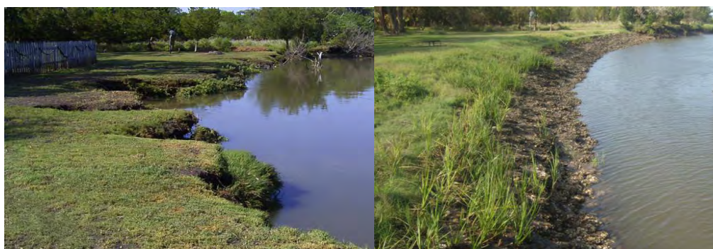
Use of oyster shell material to stabilize eroding shoreline on Sapelo Island, GA.
