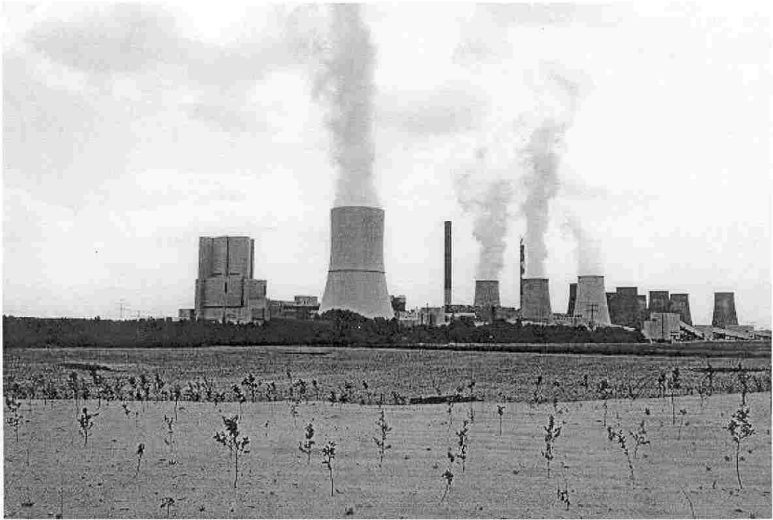
Figure 15. The power plant in Boxberg
