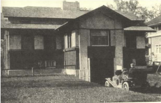
1908 Estabrook House, Tallmadge and Watson, architects.
