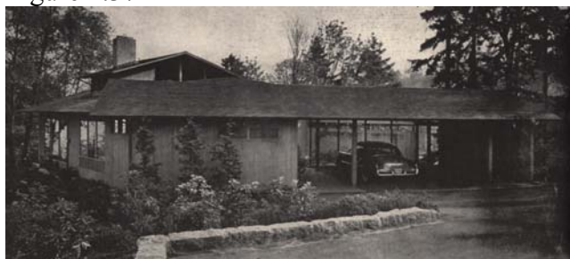
1952 carport, Pietro Belluschi, architect.
