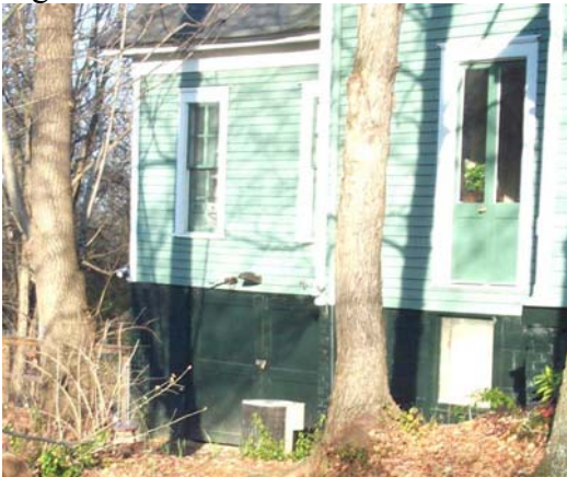
Garage constructed between foundation piers at 186 Boulevard.
