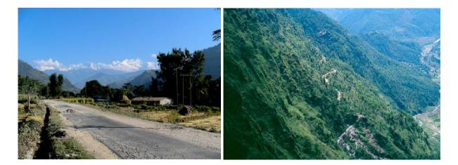
Figure 4.8 Roads in Lamjung: (a) a portion of the Dumre-Besishahar road in Dhamilikuwa VDC, and (b) a portion of the 'green road' near Baglungpani VDC—this 'environment friendly road' (no use of heavy equipments and blasting to reduce the environmental impact) is being built to promote agricultural markets and when complete it will make VDCs in western Lamjung 'market accessible.'
