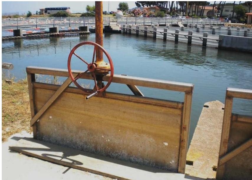
Sluice gate in the Tortoli Lagoon (Sardinia, Italy), photo ©D. Crosetti, 2011
