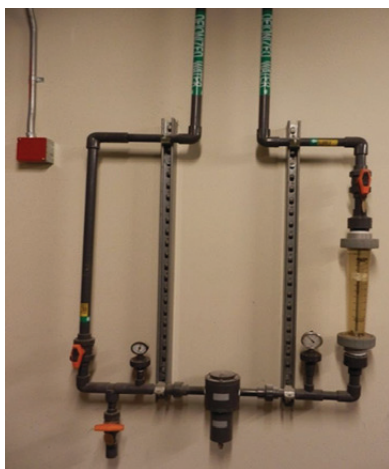
Figure 1. Parallel DI loop valves and instrumentation with 1-in branch piping connected to a 3-in main loop.
