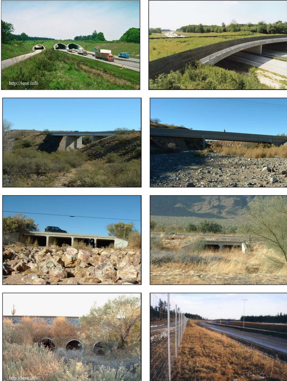
Figure 7: Road mitigation structures (top to bottom) include overpasses, bridges, culverts, and drainage pipes. Fencing (lower right) is used to guide animals to structures. (Photographs from Beier et al. 2007a).
