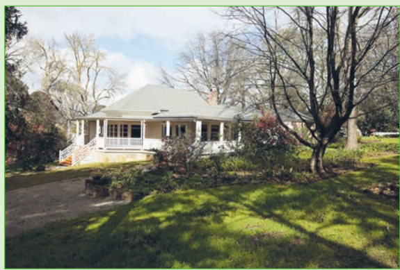
Benue Lodge before demolition. Picture: Bellholme
