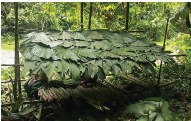
Traditional jungle hut built by a Penan, using leaves and tree poles obtained from the jungle. Photo credit: WWF-Malaysia/ Alfred Keleman
