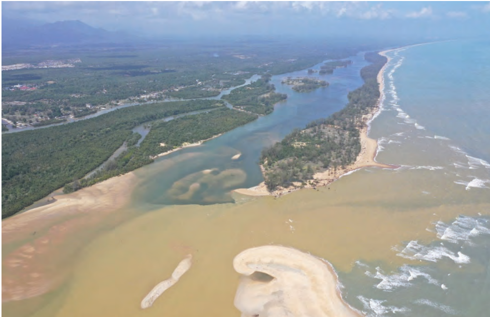
Aerial view of the Setiu lagoon, river mouth and coastal beaches. The river deepening and construction of an artificial river mouth to facilitate navigation for fishing vessels pose a threat to the wetlands ecosystem and the associated biodiversity. Photo credit: Mohamad Fadzil/WWF-Malaysia
