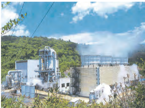
Fig. 3 Geothermal power generation facility
