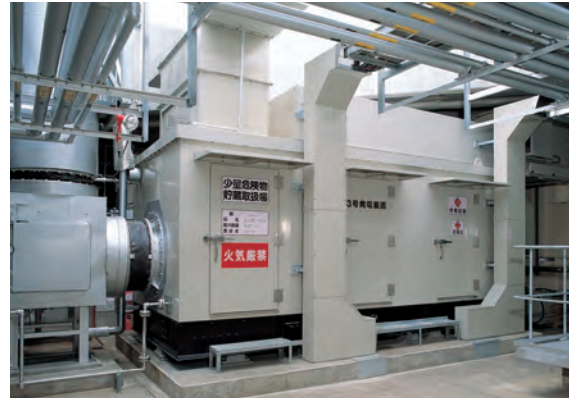
Fig. 6 Gas turbine of dual-fuel specification
