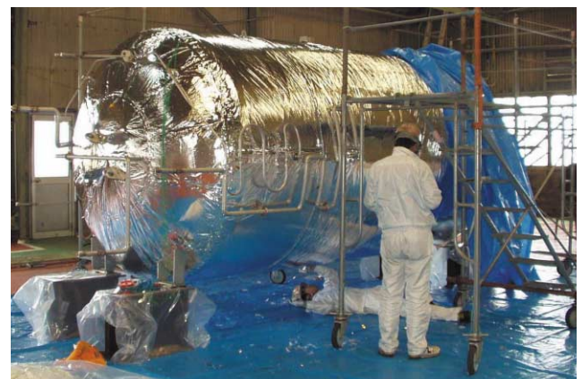
Installation of insulation
