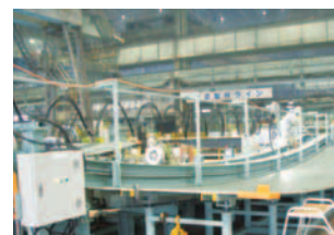
Automatic welding of 9% nickel steel tank inner wall at Harima Works
