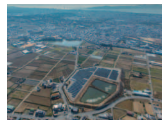
Iwaoka Photovoltaic Power Generation Station
