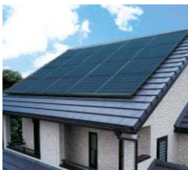
Photovoltaic Generating System for Home Use
