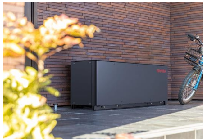
Fig. 1 The O-Uchi Kyuden System after Installation
