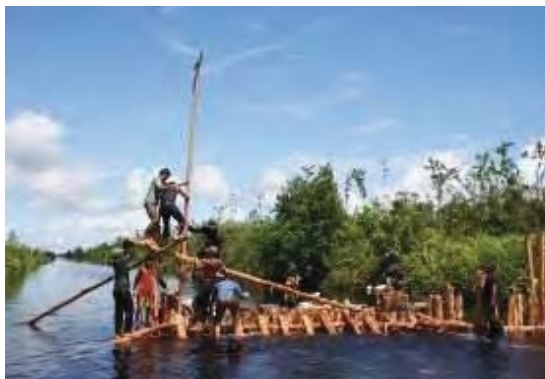
Figure 9.4: Peatland restoration Blocking of a canal in degraded peat swamp forests in Central Kalimantan, by local communities using manual traditional techniques. (Photo: Marcel Silvius, Wetlands International).
