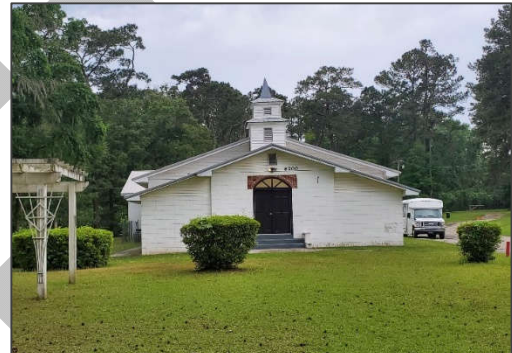
St. Phillip AME Church -Front (east) elevation-
