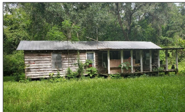
Miles-Lang Tenant House -Front (east) elevation-
