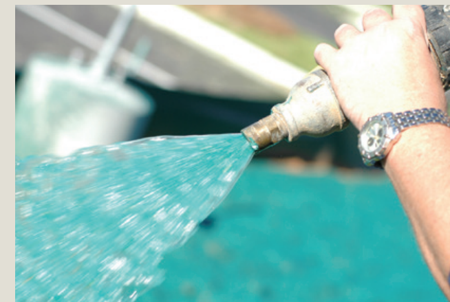
Bonded Fiber Matrix (BFM) is applied as a liquid slurry, forming a strong and durable mat of interlocking fibers to prevent soil erosion while still allowing plants to germinate and establish. ©Granite Seed Company courtesy of Profile Products
