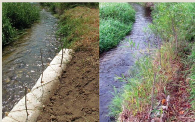
Excelsior fiber erosion control blocks used in a shoreline application with live willow stakes, pictured on the day of installation and three months later. Exterior casing is light in color compared to darker coir logs that can warm water temperatures, which can be detrimental to fish and other aquatic organisms. Functional for 3+ years, but designed to begin biodegrading during the first year as sediment and seed settle into the interior matrix. Also use in other applications such as a replacement for silt fence or for channel filter stations. ©American Excelsior Company
