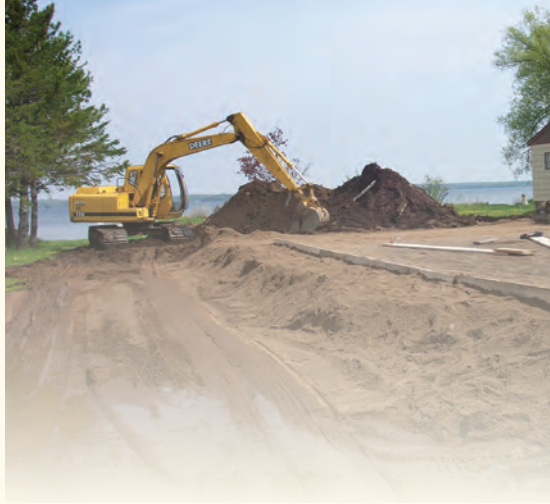
Top soil is conserved and erosion plans are in use before, during and after a land alteration.
