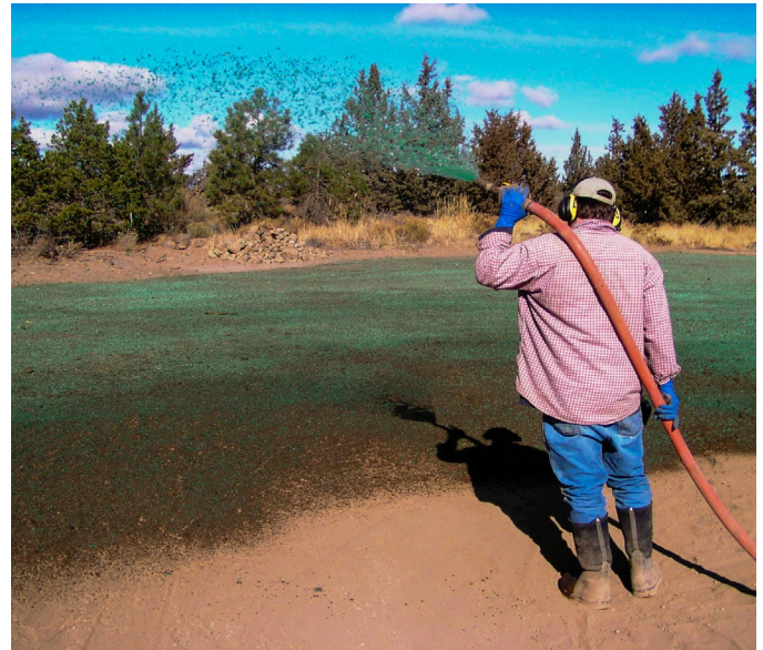
Figure 15. Hydroseeding a native plant mix including sulphur-flower buckwheat at the Deschutes National Forest Ranger District Office in Bend, OR. The broadcast hydromulch and seed was applied in fall 2011 using sulphur-flower buckwheat and other native plant seed collected about 10 miles south. The site was irrigated. Photo: C. Powers, USFS.
