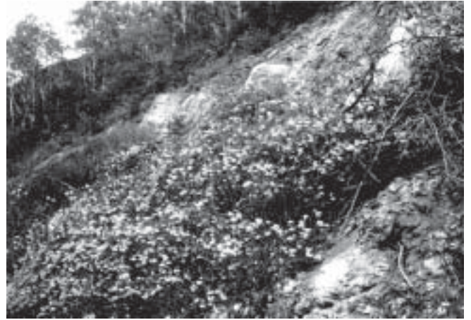
Figure 8—Crownvetch stabilizing a road cut.
