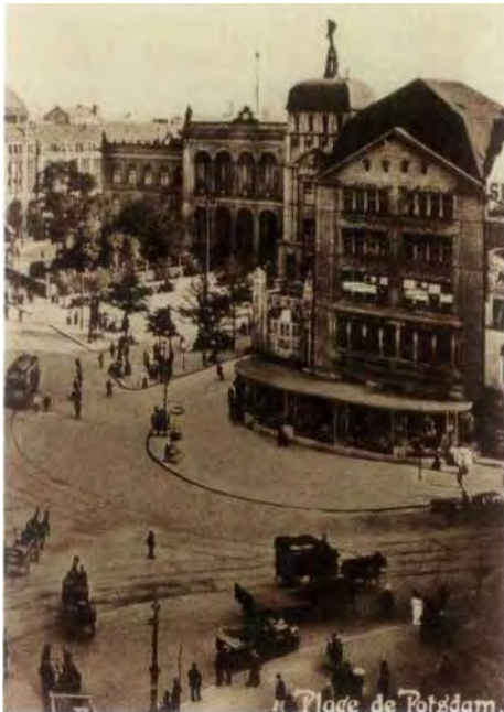
We are laying the foundations for a future built on soil fertile in tradition. The Potsdamer Platz will soon again be one of Berlin's most lively districts.
