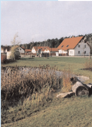
LAUBAG helps to build new villages when the local population must move as a result of the mining operations. The picture shows the Neu Geisendorf village under construction.
